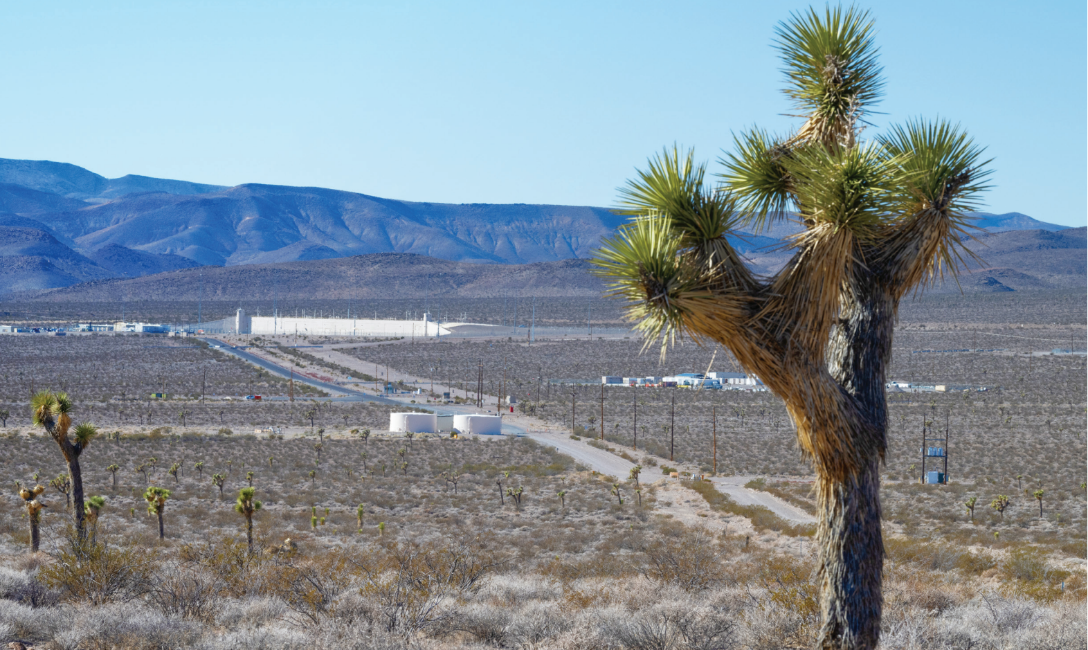
■ Originally constructed to support underground nuclear weapons tests, the Device Assembly Facility at the Nevada National Security Sites now houses NCERC and other programs that conduct important national security research.
