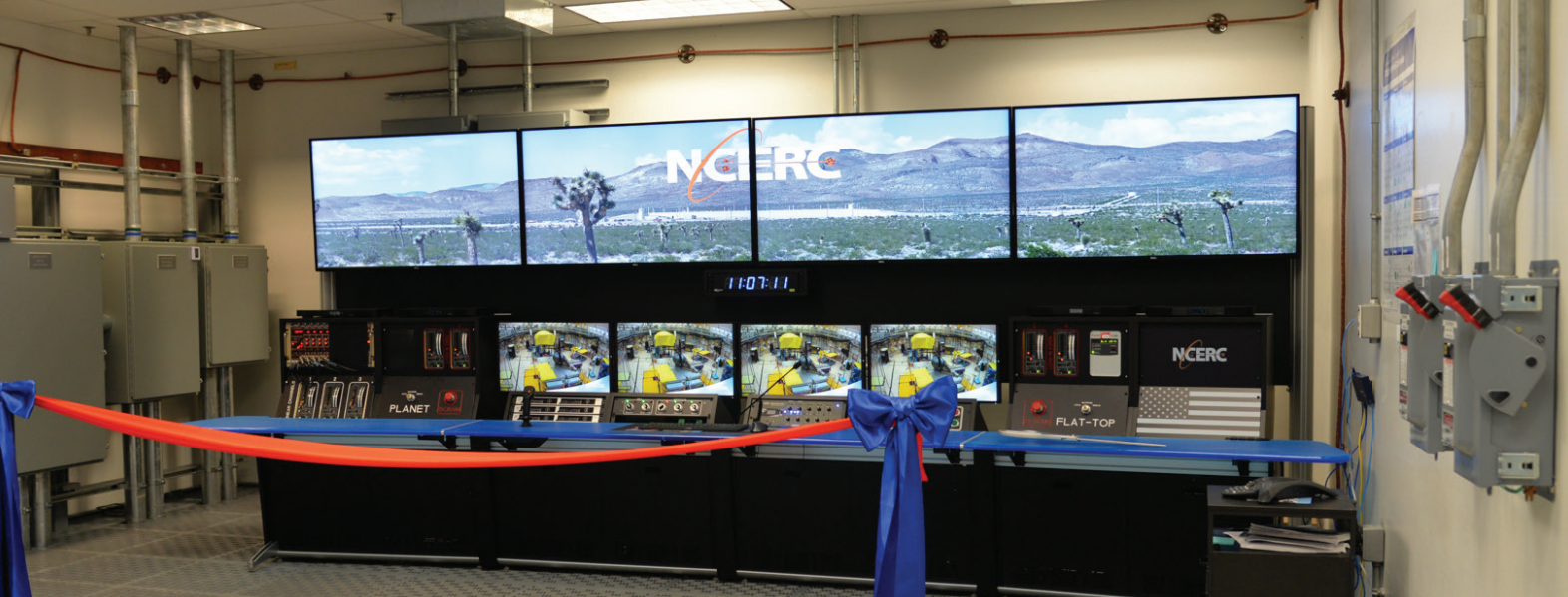
■ NCERC's Control Room 2 was upgraded in 2024 with new, state-of-the-art equipment.
