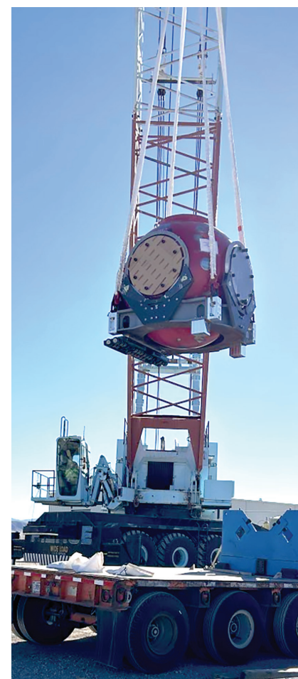
■ A 6-foot vessel is lowered 1,000 feet underground into the PULSE facility.
