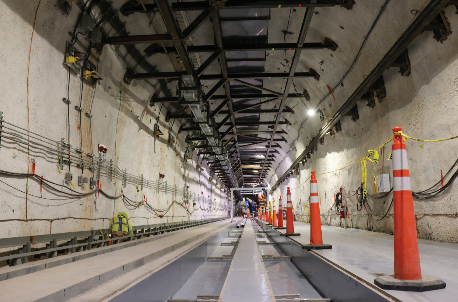
■ This tunnel will house Scorpius. Photo: NNSS
