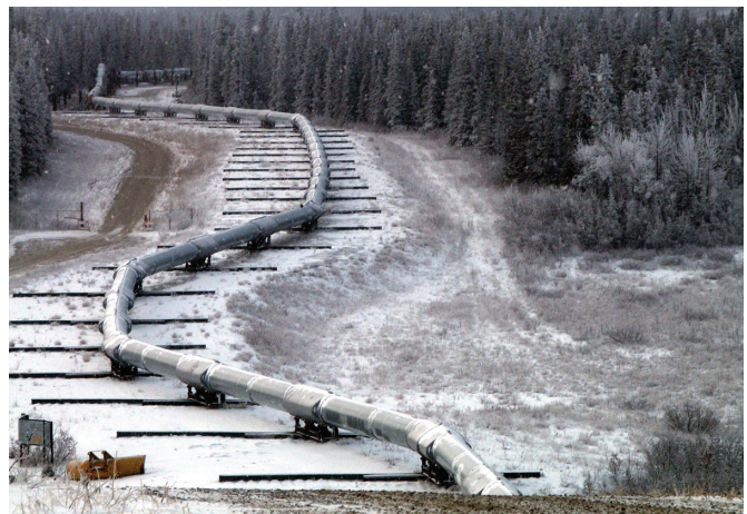
Heat pipes on the Trans-Alaska Pipeline supports prevent hot oil moving through the pipeline from melting the permafrost. Photo courtesy of the United States Geological Survey.
