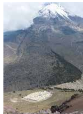
Figure 1. Photograph of the HAWC observatory that has been constructed over the last 3 years in Mexico. The site is at 13500' elevation and the mountain behind is Pico de Orizaba, the tallest mountain in Mexico at 18500'.
