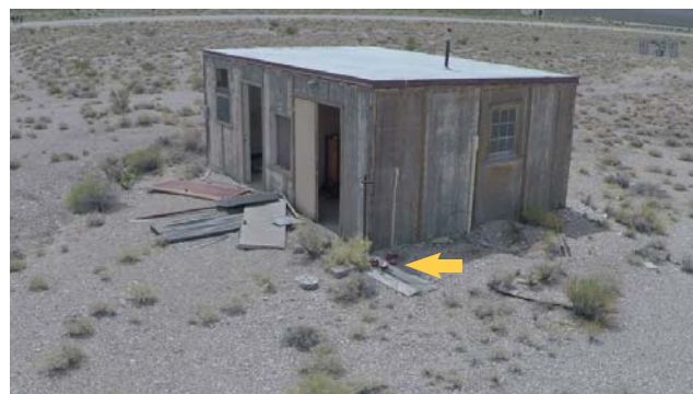
Figure 11. Image from video shot by the 3DR Solo during a source investigation demonstration. The Solo was manually flown around the building for situational awareness. Location of the sources is indicated by the yellow arrow.
