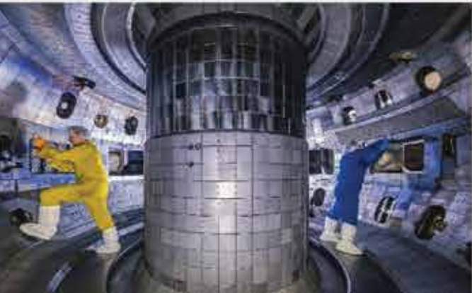
● The interior of the DIII-D tokamak, the largest operating tokamak in North America.
