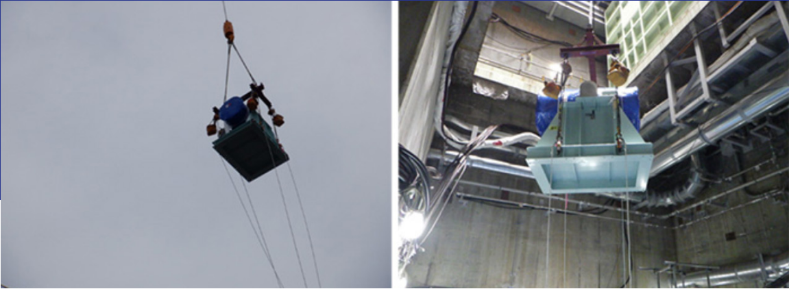
Above: IPCAS is lowered by crane through an opening in the J-MOX facility ceiling. Page 8: IPCAS is prepared for shipment at the Laboratory.
