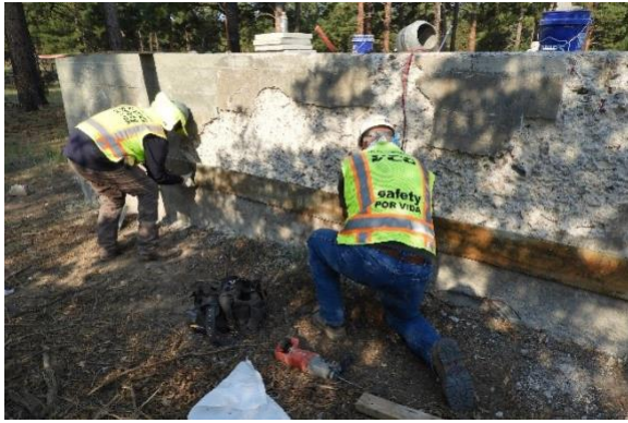
Figures 3-1 and 3-2. V-Site concrete stem walls and pad during concrete restoration in August 2020
