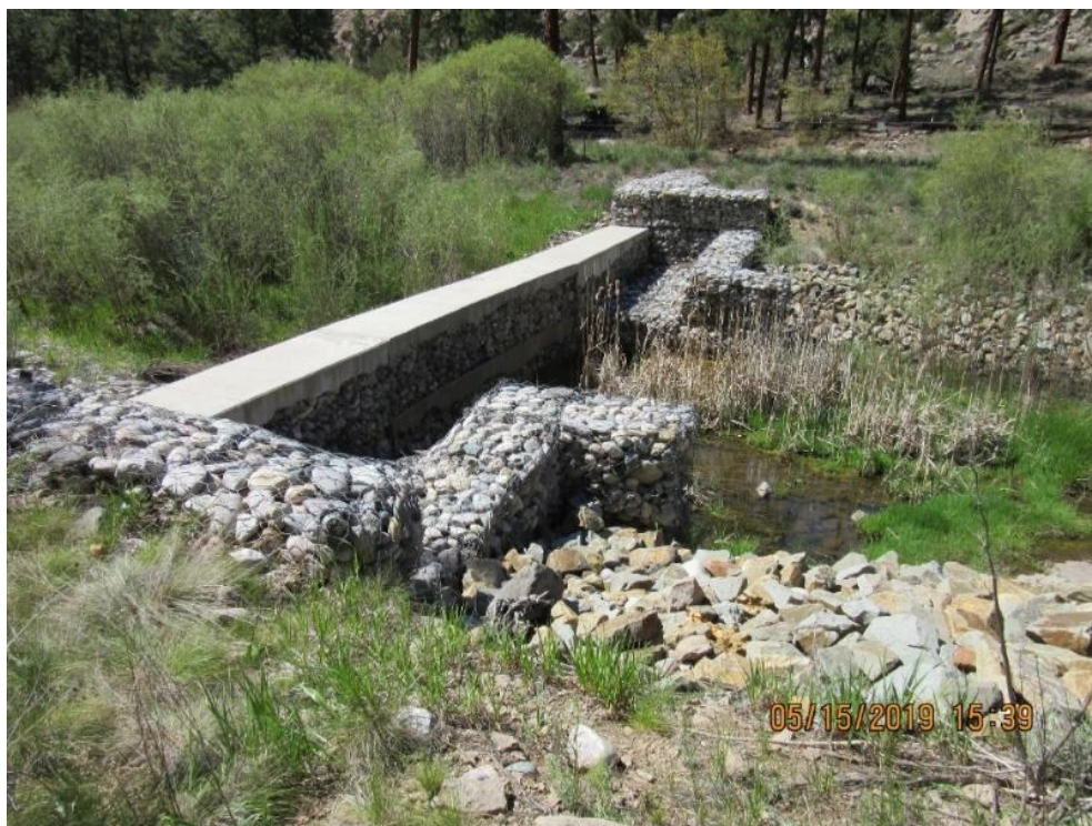
Figure 6-12. DP Canyon Grade Control Structure, looking upstream (photo taken May 2019)
