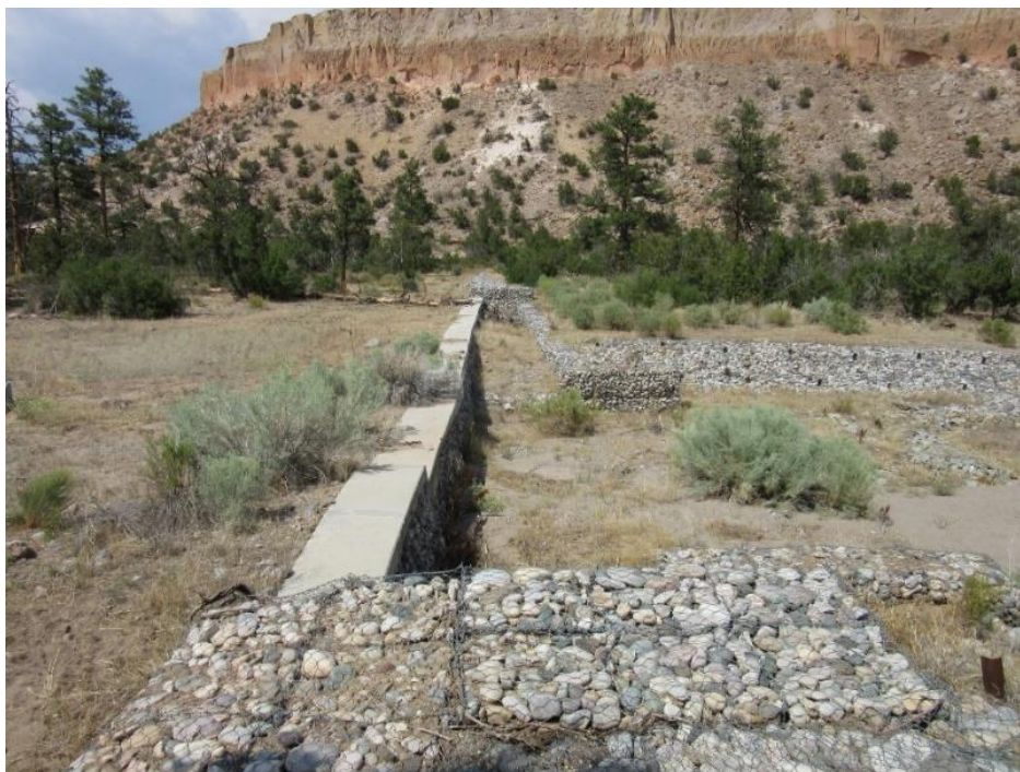
Figure 6-14. Lower Pueblo Canyon Grade Control Structure, weir crest and flow-way, looking north (photo taken August 2020)
