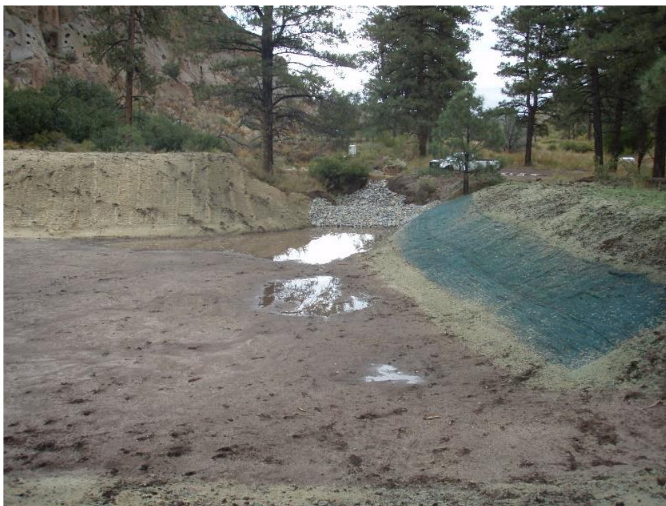
Figure 6-17. Mortandad Sediment Traps during the revitalization project in October 2014
