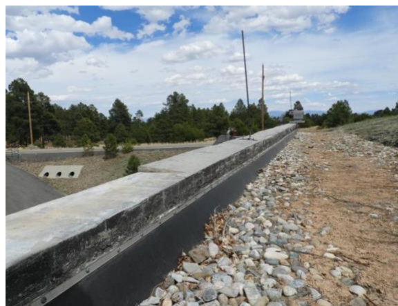
Figures 3-4 and 3-5. Gun Site parapet wall concrete cap before (left) and after (right) removal of loose concrete pieces in April 2020
