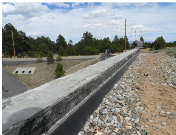
Figures 3-4 and 3-5. Gun Site parapet wall concrete cap before (left) and after (right) removal of loose concrete pieces in April 2020
