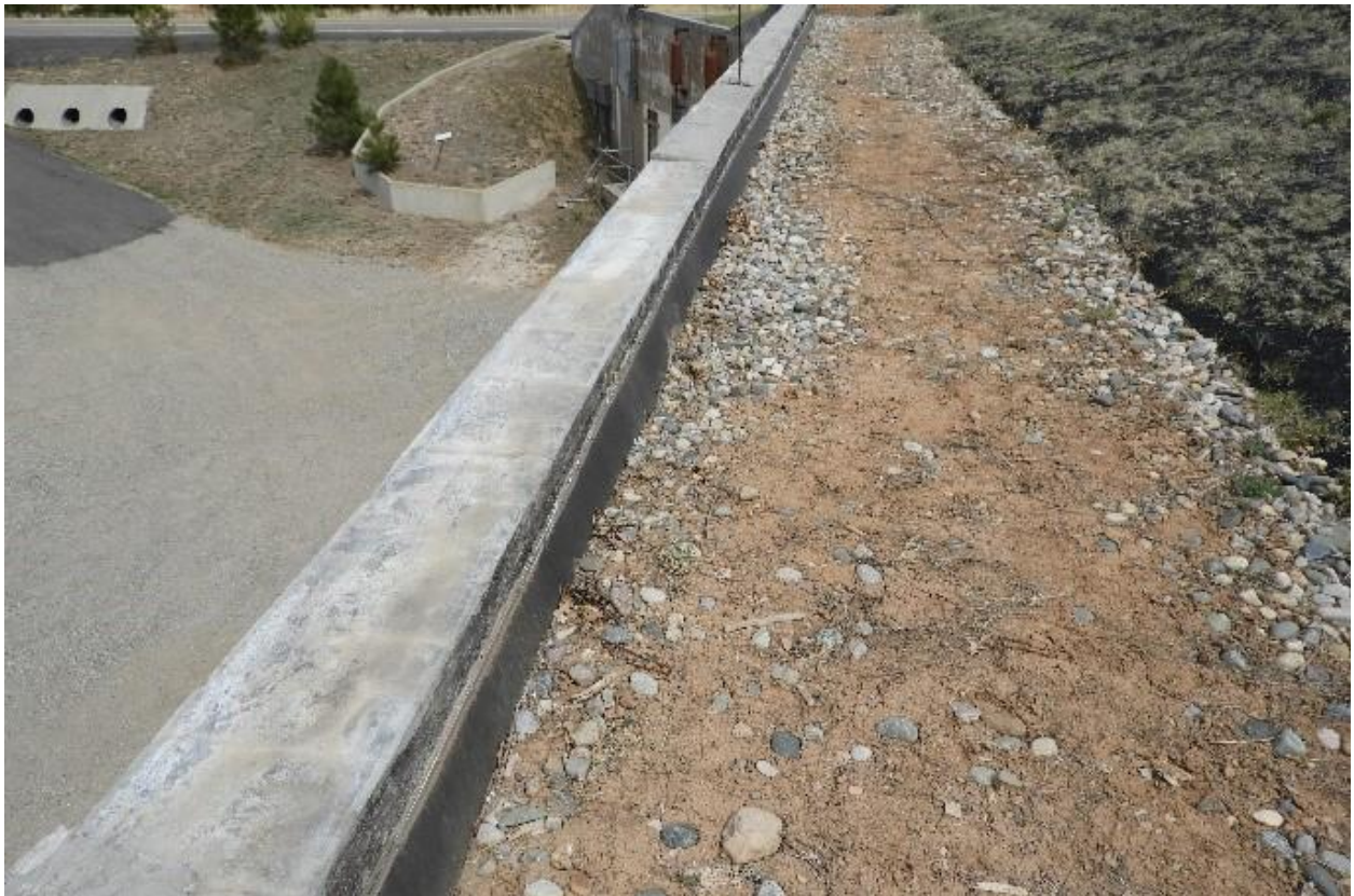
Figure 3-3. Gun Site parapet wall concrete cap after removal of loose concrete pieces in April 2020
