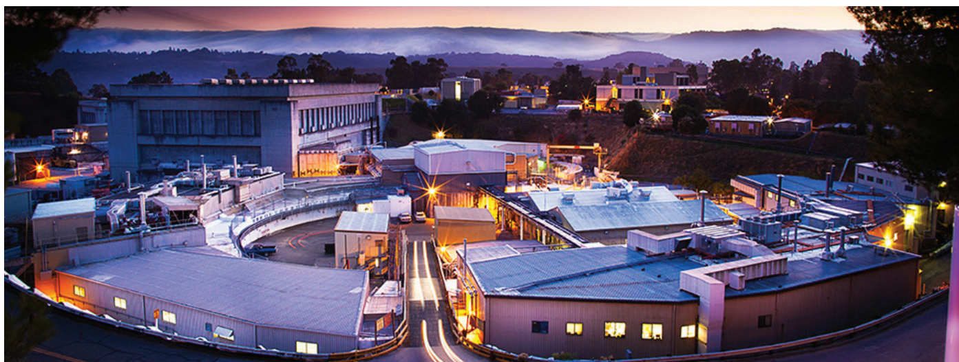
Aerial photograph of The Stanford Synchrotron Radiation Lightsource (SSRL) facility located in Menlo Park, CA.
