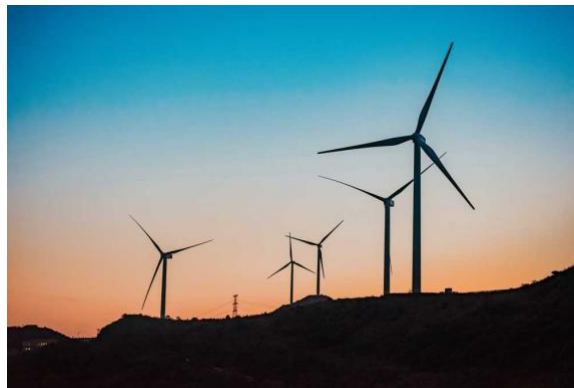
Sandia's Twistact technology proves beneficial in lowering costs, improving sustainability and reducing maintenance for next-generation direct-drive wind turbines. (Photo by Zhang Fengsheng).
